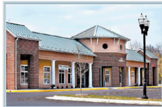
This building at 525 Amherst St. will soon house three medically-related outfits — Winchester Eye Surgery Center, Valley Home Care, and a cancer wellness center. Valley Home Care expects to be the first to take up residence by June 1. (Photo by Ginger Perry)
